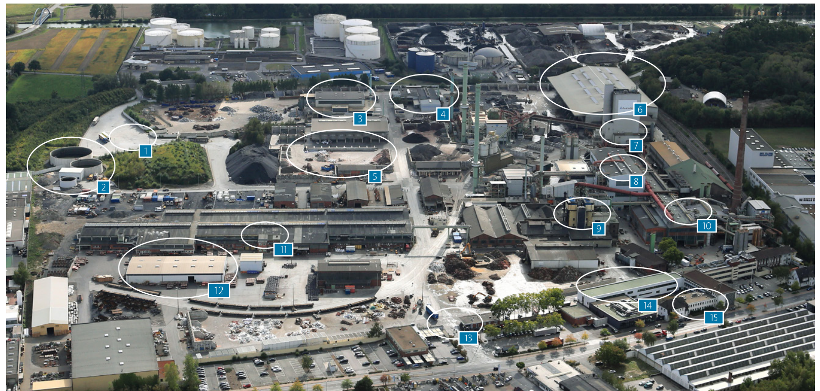
Fig. 3.1: Overview of Lünen site facilities
