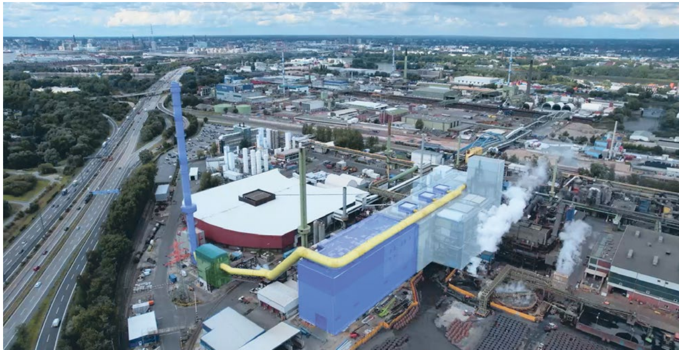
View of the new exhaust system (highlighted in color) at the Hamburg site in direct vicinity to the city
