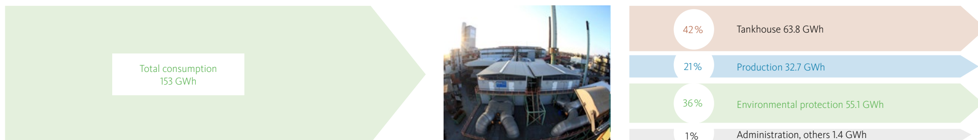
Fig. 3.17: Breakdown of energy consumption at the Lünen site
